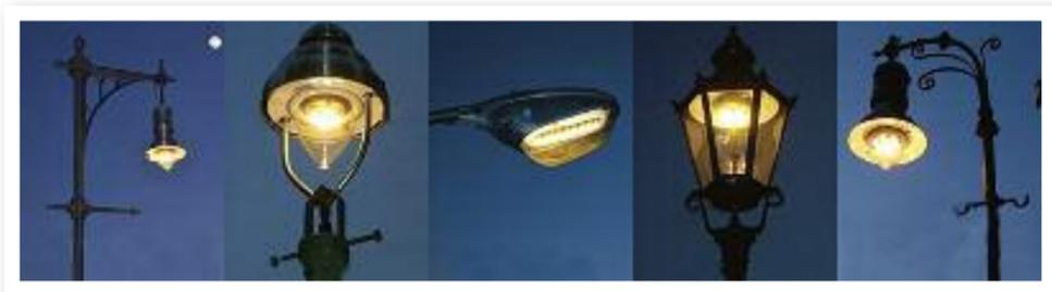
Berlin gas lamps – the five main types. **From left:** Suspended lamp with large gallows; top-piece lamp; in-line lamp; traditional lamp and suspended lamp with Wilhelminian mast PHOTOS: BERTOLD KAJATH (WWW.GASLICHT-KULTUR.DE)
